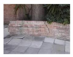
When masonry building is situated near a big tree, it is susceptible to get damaged by tree roots. Often serious damage caused by the tree roots can mean thousands of dollars in repair costs to buildings, foundations, backyards, pavements and plumbing systems.
