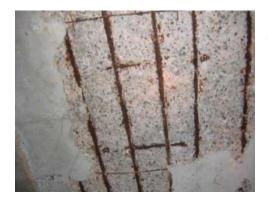
Concrete Spalling is caused when the steel reinforcing within a concrete slab begins to rust. As steel rusts it can expand 5 to 7 times its original size causing the surrounding concrete to crack and become flaky. As the steel pushes the concrete away, more water gets to the steel expediting the process. The process is often referred to as concrete cancer. For comprehensive professional report, please contact Span Consulting Engineers on (02) 9633 2280 or 0413 789 639 (M).
