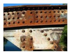
Steel is popular in construction industries for its strength, construction simplicity, time and cost benefits. Despite of its benefit, steel has a major problem of corrosion. It corrodes in about all the environments. The rate of corrosion and rust damage is depending on type of environment. For comprehensive professional report, please contact Span Consulting Engineers on (02) 9633 2280 (o) or 0413 789 639(M).
